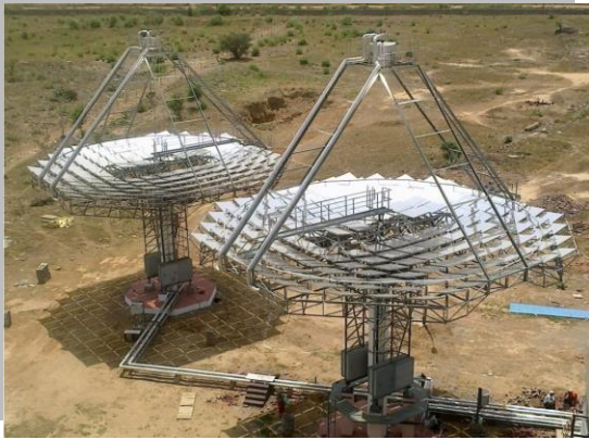
Solar Thermal Collector
